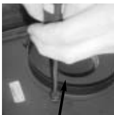
REMOVE FLUE RING
